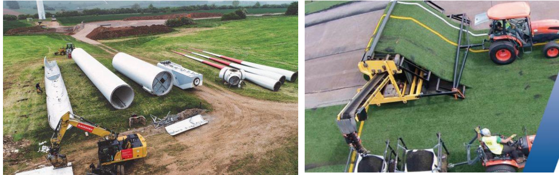
Figure 2. Removal of wind turbines (left) and artificial turf (right), where sand and rubber are automatically separated.
