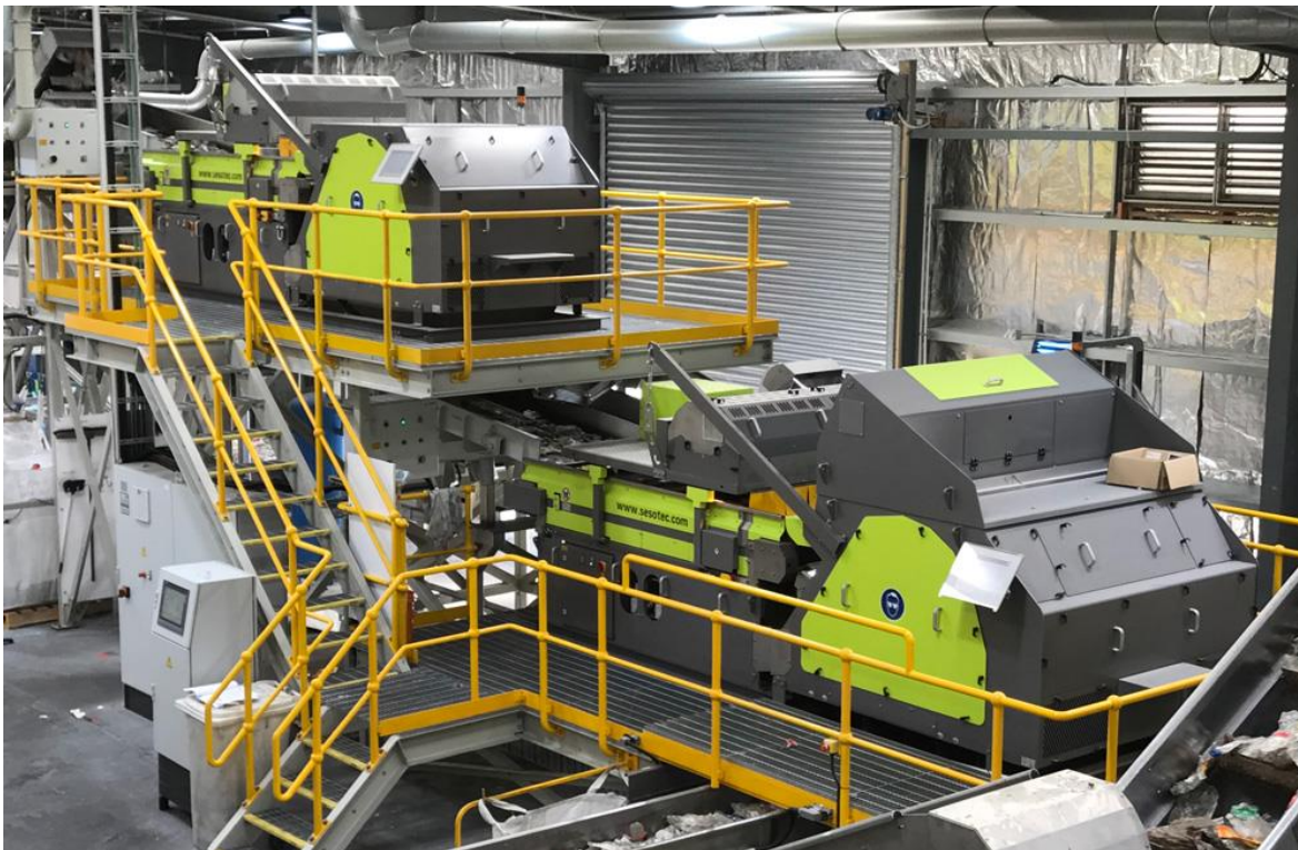
Flight Plastics installed a multi-sensor sorting line including two bottle sorters.
