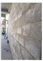
**Cape Town**, 27 February 2017. More than 15 tons of recycled, Expanded Polystyrene (EPS) have already gone into the production of 20,000 Greenlite Concrete blocks used in the new Table Bay Mall that is currently being constructed. Expected to open its doors at the end of September this year, this 65 000 m² regional shopping centre is located on a 20 ha site on the corner of the R27 (West Coast Road) and Berkshire Boulevard in the heart of the rapidly growing West Coast area.
