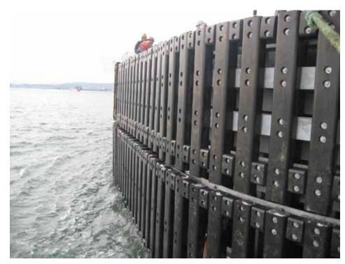
and is impervious to marine borers. The material is also designed to endure heavy impacts by absorption of energy through recoverable deflection. The company suggests that they would be well-suited for fenders in marine structures or for buildings used in coastal protection. They are also used in structural piles, bridge protection, corner fenders, navigation markers and bull rails. One of the more notable uses of the material is at the base of the Bay Bridge, linking San Francisco to Oakland.
