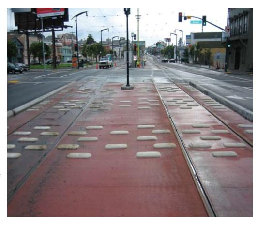
que groove system that provides for easy installation and improved adhesion for epoxy glues," with bolt holes for additional anchoring needs. The durable bumps are also "chemical and weather resistant, outlasting traditional concrete and rubber products."
